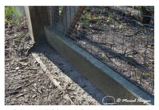
Snug fit of a gate at a wildlife fence, south of Otterlo, The Netherlands. The snug fit discourages animals from crawling under the gate.
