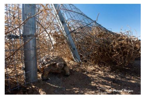
Gap at a gate associated with Mojave desert tortoise exclusion fencing, Hwy 58 near Kramer Junction, California. The gate does not have a buried component, and it had enough flex to result in permanent openings, partially as a result of tumbleweeds being blown against the fence.
