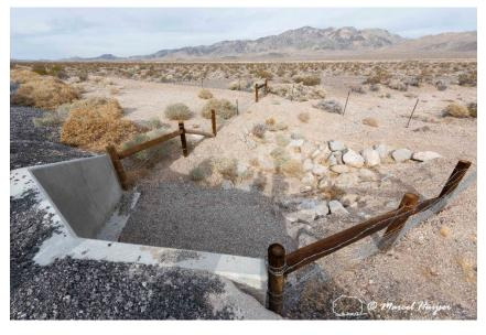
Mojave desert tortoise fencing connected to a concrete box culvert (lower left), US Hwy 95 (MP 125 NB) near Indian Springs, Nevada. Note that the fences angle from the property boundary towards the culvert to funnel the animals towards the culvert. Also note that the property boundary fence continues through the wash (this property boundary fence is not a barrier to Mojave desert tortoises).
