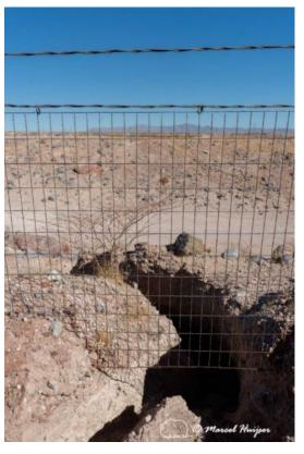
Mojave desert tortoise fencing with soil erosion, I-11, near Boulder City, Nevada. Note that the animals may now move in the erosion gully under the fence. Also note that the fence appears to have only been dug 6 inches into the ground rather than the recommended minimum 12 inches.
