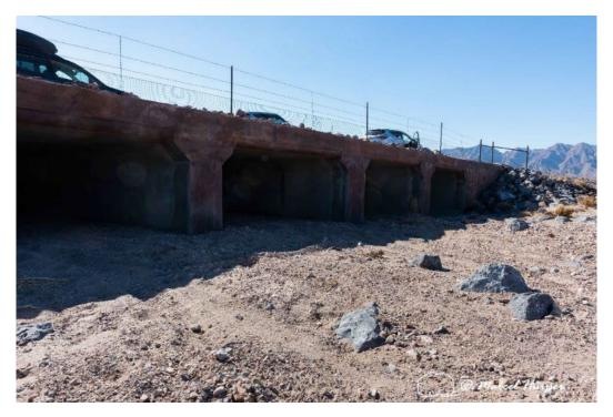
Riprap filled in with finer rocks and sand, in front of culverts to reduce erosion, I-11, near Boulder City, Nevada. This does not appear to be a barrier to Mojave desert tortoises.
