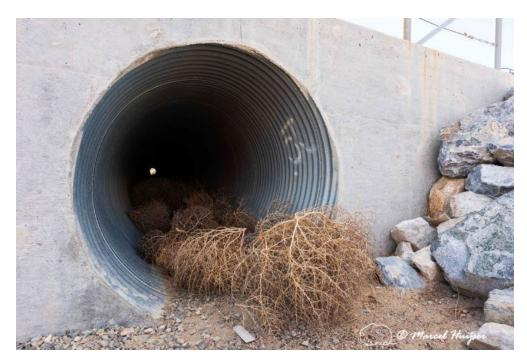
Culvert primarily constructed for hydrology, but the culvert may also allow for passage by Mojave desert tortoises I-15 near Barstow, California. However, this culvert is blocked by tumbleweed.
