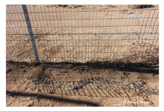
Mojave desert tortoise exclusion fence, Hwy 58 near Kramer Junction, California. Here the fence is angled towards the safe side of the fence (not the roadside), presumably because of rocky soil. Also note that the section of the fence that lies on the ground should be buried up with to 4 inches of rocks and soil on top, leaving a barrier height of 22-24 inches above the ground level.
