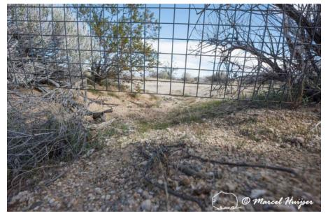
Gap under Mojave desert tortoise exclusion fence, USA Aerospace Highway (Hwy 14), near Inyokern, California. The small mesh size may pose a greater risk to small animal species (lizards, snakes) getting stuck and dying. Small mesh sizes are also more likely to catch sediment. Note that this fence is not buried at all. Mojave desert tortoise fencing should be buried at least 12 inches deep.
