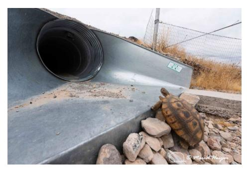
Close-up with adult tortoise model at a corrugated metal culvert (Corrugated Metal Pipe (CMP), US Hwy 93 (MP 58 NB) near Overton, Nevada. Note that the height of the drop-off at the outflow of the culvert is likely a barrier for smaller size tortoises. While adult tortoises have been observed to pass through this culvert, regular monitoring and maintenance to address the effects of erosion can help keep a culvert passable by a both adult and juvenile tortoises.
