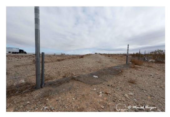
Flattened and destroyed gate at a vehicle access point associated with a Mojave desert tortoise fence, I-15 near Barstow, California. Here the fence has, or had, a gate for a dirt road, but the fence was flattened by vehicles. This suggests that gates that require people to get out of the vehicles to open
