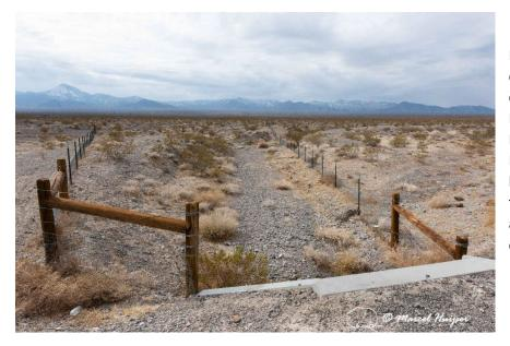
Funnel fencing for Mojave desert tortoise and a box culvert (foreground), US Hwy 95 (MP 126.5 SB) near Indian Springs, Nevada. Note that the fence on the left is on higher ground, on top of the bank of the wash, and not within the wash or on the bank.
