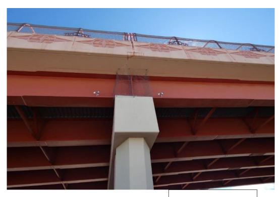
Wire mesh and metallic flashers installed to discourage raven nesting on Snow Mountain Overpass, U.S. 95, Las Vegas, Nevada.
