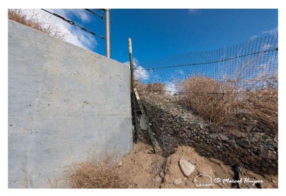
Mojave desert tortoise fencing connected to a culvert, I-15 near Barstow, California. Here debris (rocks, sand) has built up against the fence, threatening its integrity.
