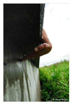
Concrete barrier wall integrated into the roadbed, with overhang, designed and implemented to keep reptiles, amphibians and small mammals off a highway, U.S. 441, Paynes Prairie Ecopassage, south of Gainesville, Florida, USA. Depending on design and construction, this type of barrier might not affect landscape aesthetics as experienced from the road.
