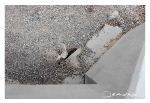
Erosion along a concrete pathway leading up to a concrete box culvert, US Hwy 95 (MP 127.5 NB) near Indian Springs, Nevada. The riprap is filled with finer sediments that allows Mojave desert tortoises to access the culvert. However, it appears that the finer sediments are washing out and resulting in cavities that could trap Mojave desert tortoises.
