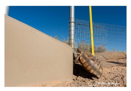
Mojave desert tortoise fencing connected to the wingwall of a culvert, Hwy 58 near Kramer Junction, California. While the connection between the fence and wingwall is tight and should not allow Mojave desert tortoises to access the fenced road corridor, the effective height at the connection is only about 11 inches instead of the recommended 22-24 inches. The fence material should have been continued until the point where the wingwall has a height of 22-24 inches.
