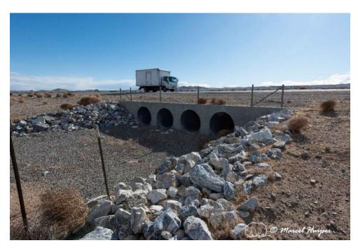
Mojave desert tortoise fencing leading up to culverts primarily designed for hydrology, I-15 near Barstow, California. Note that the fence does not physically connect to the structure and that riprap (rocks) fills the gap. However, it would have been better to leave no gap in the fence and have the fence continue on top of the bank above the boulders.
