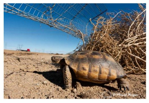
Gap under a gate associated with Mojave desert tortoise exclusion fencing, Hwy 58 near Kramer Junction, California. The gate does not have a buried component, and it had enough flex to result in permanent openings, partially as a result of tumbleweeds being blown against the fence.
