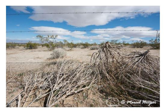
Dead vegetation has blown against the Mojave desert tortoise fence, reducing the barrier effect of the fence to keep tortoise from accessing the highway, Aerospace Hwy, Hwy 14 near Inyokern, California.
