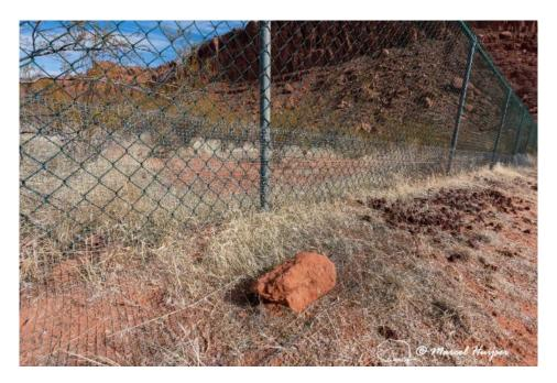
Mojave desert tortoise exclusion fence, St. George, Utah. Normally, the fence should be buried, but here it is above ground, held down by rocks. Note: the section of the fence that lies on the soil should face the safe side (habitat side) of the fence (not the roadside). Also note that the section of the fence that lies on the ground should be buried up with to 4 inches of rocks and soil on top, leaving a barrier height of 22-24 inches above the ground level.
