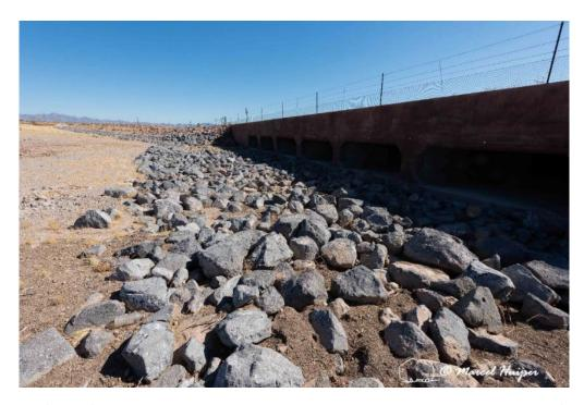
Riprap in front of culverts to reduce erosion, I-11, near Boulder City, Nevada. While beneficial to combatting erosion and sedimentation issues, the size and placement of the riprap most likely results in a substantial barrier to Mojave desert tortoises.
