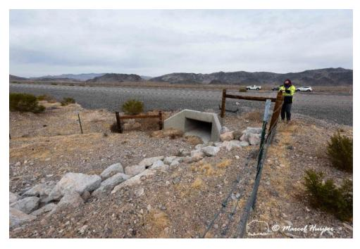
Mojave desert tortoise fencing and a concrete box culvert, US Hwy 95 (MP 127.5 SB) near Indian Springs, Nevada. Note that the fence on the near side is located on top of the bank of the desert wash, and not in the wash or on the bank.
