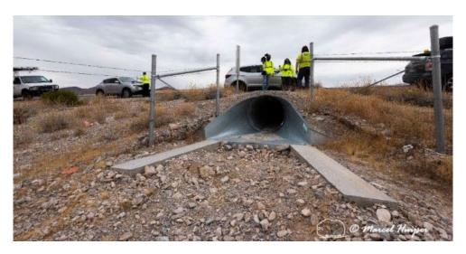
Mojave desert tortoise fence connected to a corrugated metal pipe (culvert) (CMP) with concrete pathways on both sides for Mojave desert tortoises, US Hwy 93 (MP 58 NB) near Overton, Nevada. Note that erosion resulted in a drop-off at the outflow of the culvert and this is likely a barrier to juvenile tortoises. While this culvert is passable for Mojave desert tortoises, improvements can be made by reducing the height of the drop-off.
