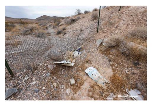
Mojave desert tortoise exclusion fencing across a desert wash with sedimentation at the fence, US Hwy 93 (MP 58 NB) near Overton, Nevada. The sedimentation reduces the effective height of the fence, and it may eventually threaten the integrity of the fence. Also note that the fence material has been cut in multiple overlapping segments to allow for the change in angle because of the change in slope (see next image for details).
