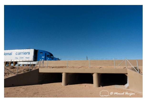
Culverts, primarily designed for hydrology, but also for Mojave desert tortoises, Hwy 58 near Kramer Junction, California. There is no erosion or sedimentation at this approach that would constitute a barrier to tortoises. However, having one open structure, not separated by dividing walls, would likely be better for wildlife use in general.
