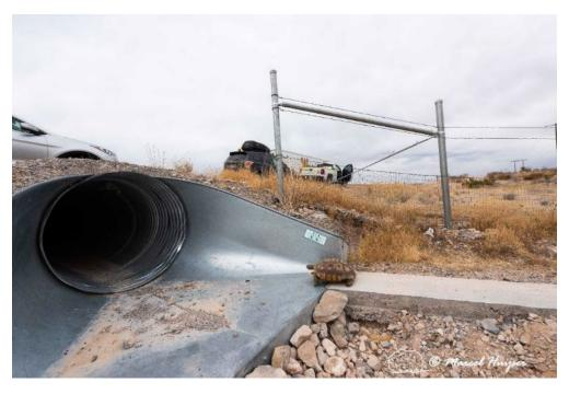
An adult tortoise model demonstrates how this concrete pathway may allow access to the culvert entrance, US Hwy 93 (MP 58 NB) near Overton, Nevada. As noted above, the drop-off at the outflow of the culvert is a potential barrier to juvenile tortoises.
