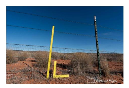
Mojave desert tortoise fencing, St. George, Utah. This fence has a mesh size that is 1 inch wide and 2 inches tall, the fence material is 20 inches above the ground, and it is attached with hog rings to three smooth strands of wire (at 4, 12, and 20 inches above the ground). There are two additional smooth wires above the fence material. Presumably, the fencing material is dug into the ground, about 16 inches deep.
