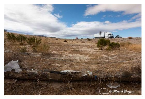
Mojave desert tortoise fencing installed across a low lying area, along I-15 near Barstow, California. Here debris (rocks, sand, garbage) has built up against the fence because water runs down the slope against the fence.
