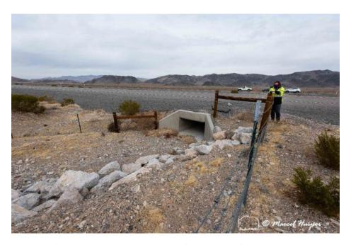
Mojave desert tortoise fence and a culvert US Hwy 95 (MP 127.5 SB) near Indian Springs, Nevada. Riprap stabilizes the slope between the fence and the culvert. Mojave desert tortoises that follow the fence cannot easily access the culvert; they would have to navigate the riprap on the slope first. Design and construction of culverts, fences, and measures aimed at erosion control should ensure that tortoises can easily access the culvert, including when they follow the fence.
