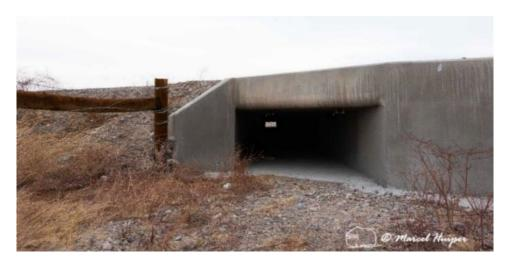
Mojave desert tortoise fence and a culvert with concrete pathways leading up to the entry, US Hwy 95 (MP 121.6 SB) near Indian Springs, Nevada. This inflow shows no noticeable erosion; Mojave desert tortoises of any size can easily access this culvert across the entire width of the culvert.
