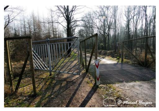
Horse swing gate, Heugterdijk, Weerterbos, near Maarheze, The Netherlands. The center of the metal swing gate is set at an angle so that gravity automatically brings the metal gate in line with the fence. Here the gate is in the process of closing.
