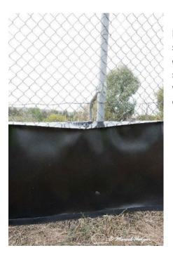
Solid plastic fencing for small animal species attached to a chain-link fence designed for larger wildlife species, M79 motorway, south of Harcourt, Victoria, Australia. However, in arid ecosystems, erosion and sedimentation processes may be a substantial problem for this design as it is not permeable to water and fine sediments and solid barriers may also be more easily damaged by high winds.
