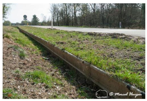
Polymer wall for amphibians integrated into the roadbed, The Netherlands. This type of barrier does not affect landscape aesthetics as experienced from the road. The design also allows for tortoises to exit the road anywhere by tumbling down the barrier. The height may have to be adjusted to prevent large adult desert tortoises from climbing over the barrier while not posing any threat of injury to tortoises that may fall over the barrier.
