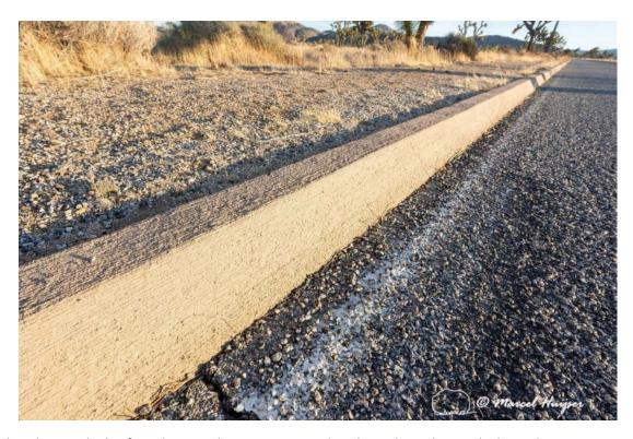
Curb to keep vehicles from leaving the pavement and parking along the roadside, Joshua Tree National Park, California. Denying vehicles access to the road shoulder can be combined with habitat restoration. The rough surface of the curb is to potentially allow Mojave desert tortoises to escape from the road.
