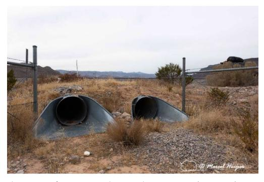
Mojave desert tortoise fencing connected to twin culverts, US Hwy 93 (MP 69.5 NB) near Overton, Nevada. The fencing would be a more effective barrier if it was continued above the culvert without any gap in the fence.
