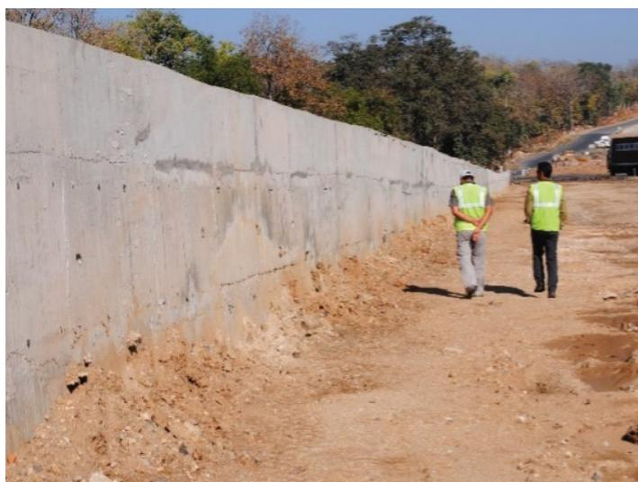
Figure 42. A dual-purpose reinforced concrete sound and elephant barrier wall in India.
