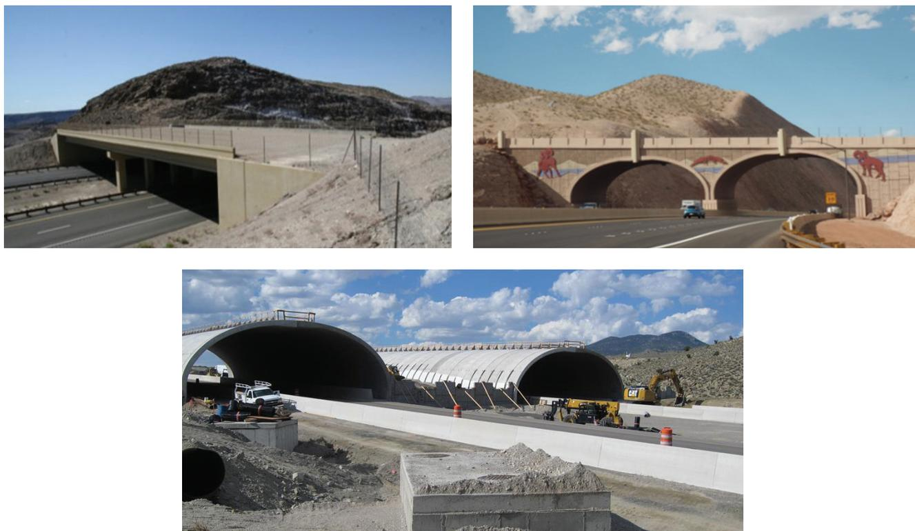
Figure 25. Overpass design types, including girder bridge (top left); concrete arch (top right); retrofit metal-plate arch on an existing highway (bottom). All examples from the USA.
