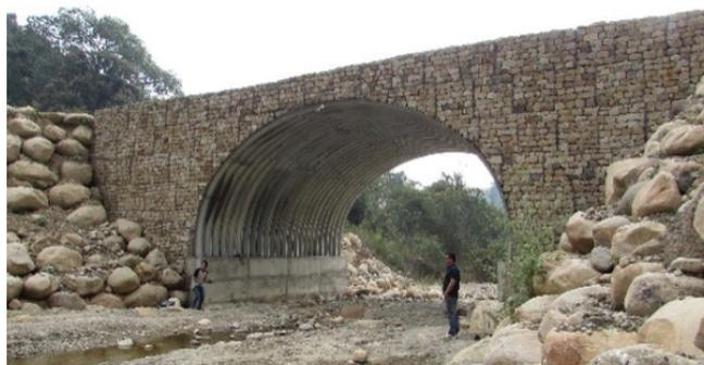
Figure 5. Minor bridge arch underpass in Bhutan.
