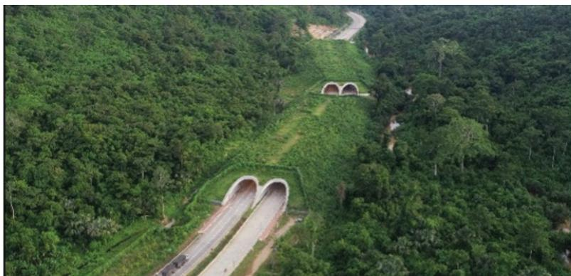
Figure 23. Highway 304 wildlife overpass in Thailand comprised of two twin 16 m precast arches extending 0.17 and 0.25 km spanning the highway.
