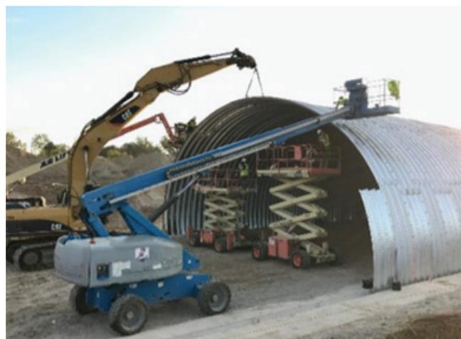
Figure 18. Metal-plate arch underpass in southern Bhutan (left); underpass being erected (right).
