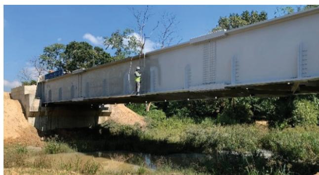
Figure 15. Single-span girder minor bridges that serve as Asian elephant underpasses, including a highway bridge in Nepal (left) and a railway bridge in Bangladesh (right), both under construction.
