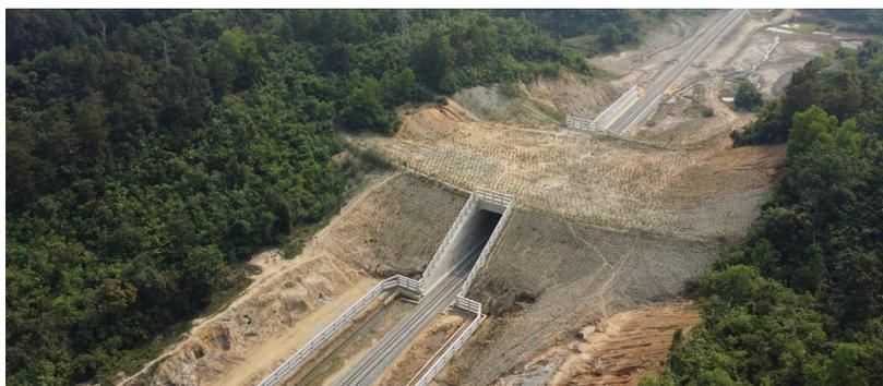
Figure 24. Newly constructed elephant overpass spanning a new railway line in southeastern Bangladesh (top left); with backfilling around the structure (top right); to reconnect the excavated elephant travel corridor along the ridgeline (bottom).
