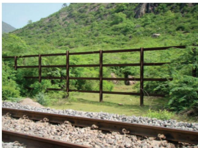
Figure 38. Applications of railway track elephant barrier fencing with two horizontal track bars (left) and four horizontal track bars in Posita, Jharkhand, India (right).
