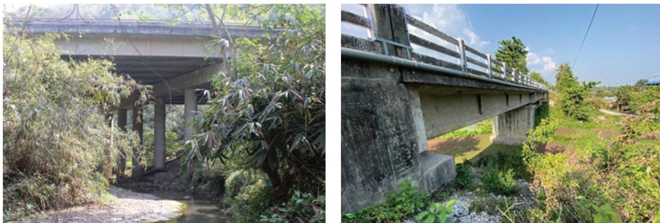
Figure 19. Major bridge underpass designed specifically for Asian elephant passage along the Sixiao Expressway in South Yunnan, China (left); dual-use structure spanning a river in southern Nepal (right).
