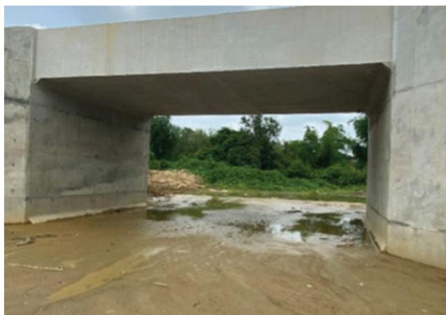
Figure 17. A 6.2 m wide × 4.7 m high underpass on Bhutan NH2 used by Asian elephants (left); reinforced concrete box culvert Asian elephant underpass (10 m wide × 5 m high × 6.9 m long) along a railway in southeast Bangladesh (right).
