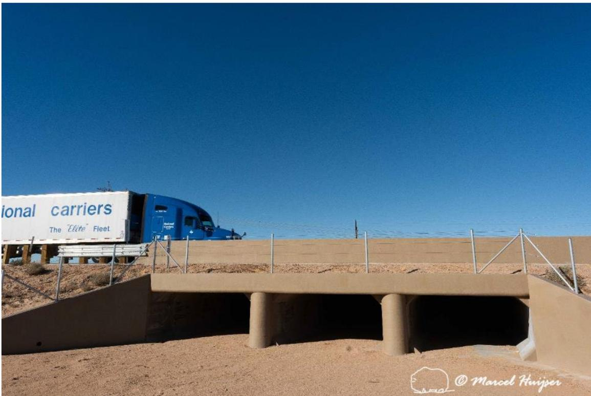
Culverts, primarily designed for hydrology, but also for Mojave desert tortoises, Hwy 58 near Kramer Junction, California. There is no erosion or sedimentation at this approach that would constitute a barrier to tortoises. However, having one open structure, not separated by dividing walls, would likely be better for wildlife use in general.
