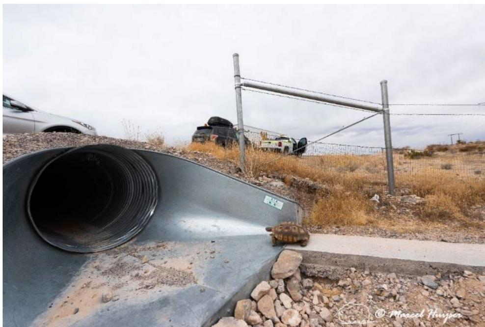
An adult tortoise model demonstrates how this concrete pathway may allow access to the culvert entrance, US Hwy 93 (MP 58 NB) near Overton, Nevada. As noted above, the drop-off at the outflow of the culvert is a potential barrier to juvenile tortoises.
