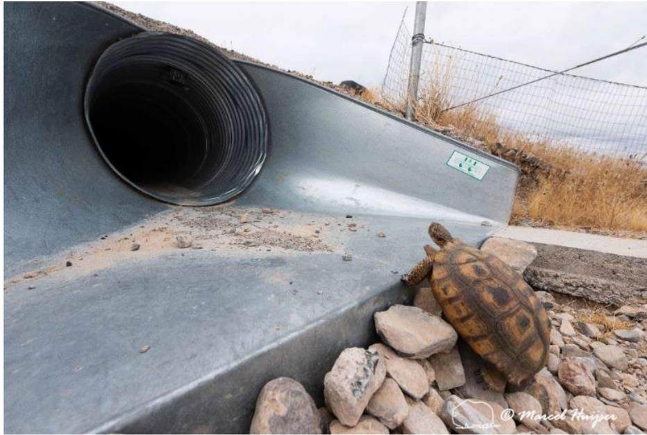
Close-up with adult tortoise model at a corrugated metal culvert (Corrugated Metal Pipe (CMP), US Hwy 93 (MP 58 NB) near Overton, Nevada. Note that the height of the drop-off at the outflow of the culvert is likely a barrier for smaller size tortoises. While adult tortoises have been observed to pass through this culvert, regular monitoring and maintenance to address the effects of erosion can help keep a culvert passable by a both adult and juvenile tortoises.
