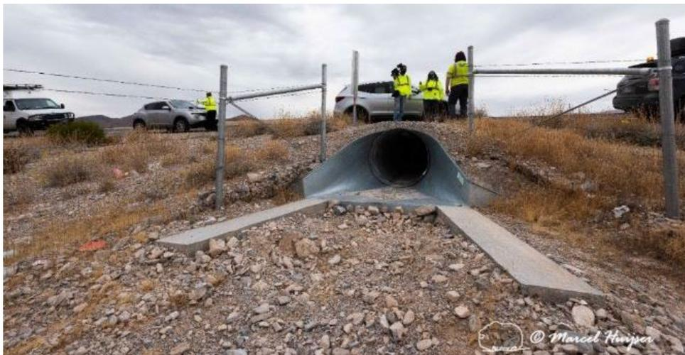
Mojave desert tortoise fence connected to a corrugated metal pipe (culvert) (CMP) with concrete pathways on both sides for Mojave desert tortoises, US Hwy 93 (MP 58 NB) near Overton, Nevada. Note that erosion resulted in a drop-off at the outflow of the culvert and this is likely a barrier to juvenile tortoises. While this culvert is passable for Mojave desert tortoises, improvements can be made by reducing the height of the drop-off.
