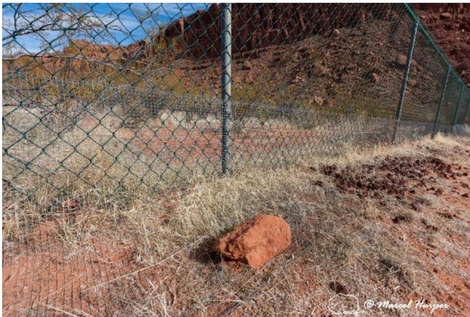
Mojave desert tortoise exclusion fence, St. George, Utah. Normally, the fence should be buried, but here it is above ground, held down by rocks. Note: the section of the fence that lies on the soil should face the safe side (habitat side) of the fence (not the roadside). Also note that the section of the fence that lies on the ground should be buried up with to 4 inches of rocks and soil on top, leaving a barrier height of 22-24 inches above the ground level.
