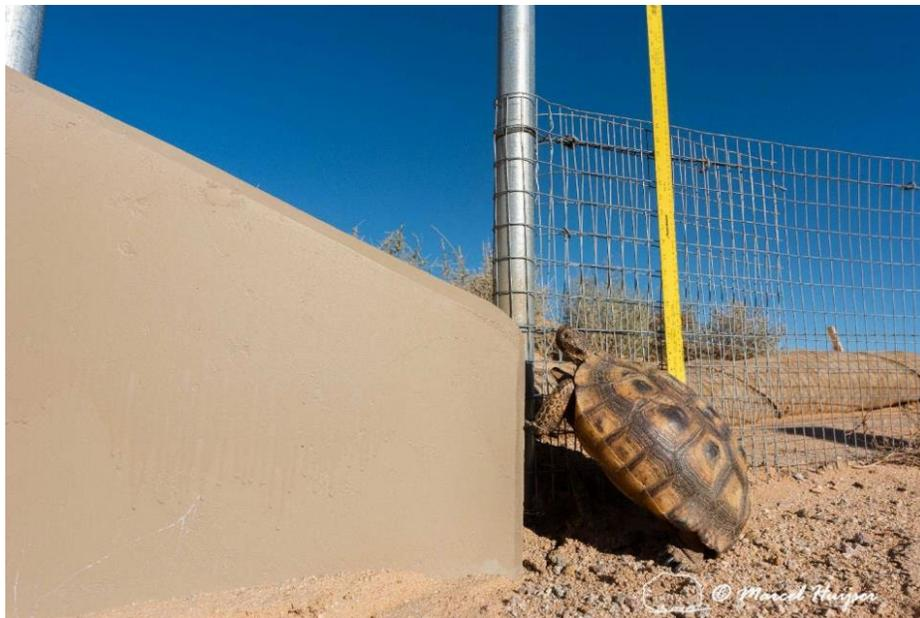
Mojave desert tortoise fencing connected to the wingwall of a culvert, Hwy 58 near Kramer Junction, California. While the connection between the fence and wingwall is tight and should not allow Mojave desert tortoises to access the fenced road corridor, the effective height at the connection is only about 11 inches instead of the recommended 22-24 inches. The fence material should have been continued until the point where the wingwall has a height of 22-24 inches.
