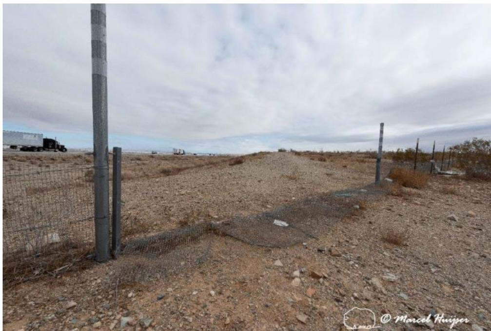
Flattened and destroyed gate at a vehicle access point associated with a Mojave desert tortoise fence, I-15 near Barstow, California. Here the fence has, or had, a gate for a dirt road, but the fence was flattened by vehicles. This suggests that gates that require people to get out of the vehicles to open
