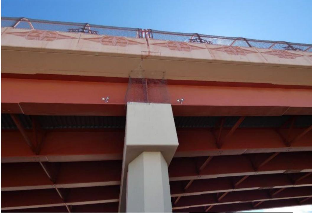
Wire mesh and metallic flashers installed to discourage raven nesting on Snow Mountain Overpass, U.S. 95, Las Vegas, Nevada.
