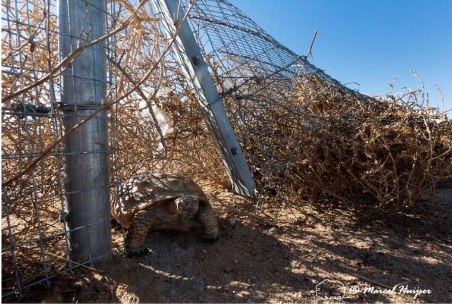
Gap at a gate associated with Mojave desert tortoise exclusion fencing, Hwy 58 near Kramer Junction, California. The gate does not have a buried component, and it had enough flex to result in permanent openings, partially as a result of tumbleweeds being blown against the fence.
