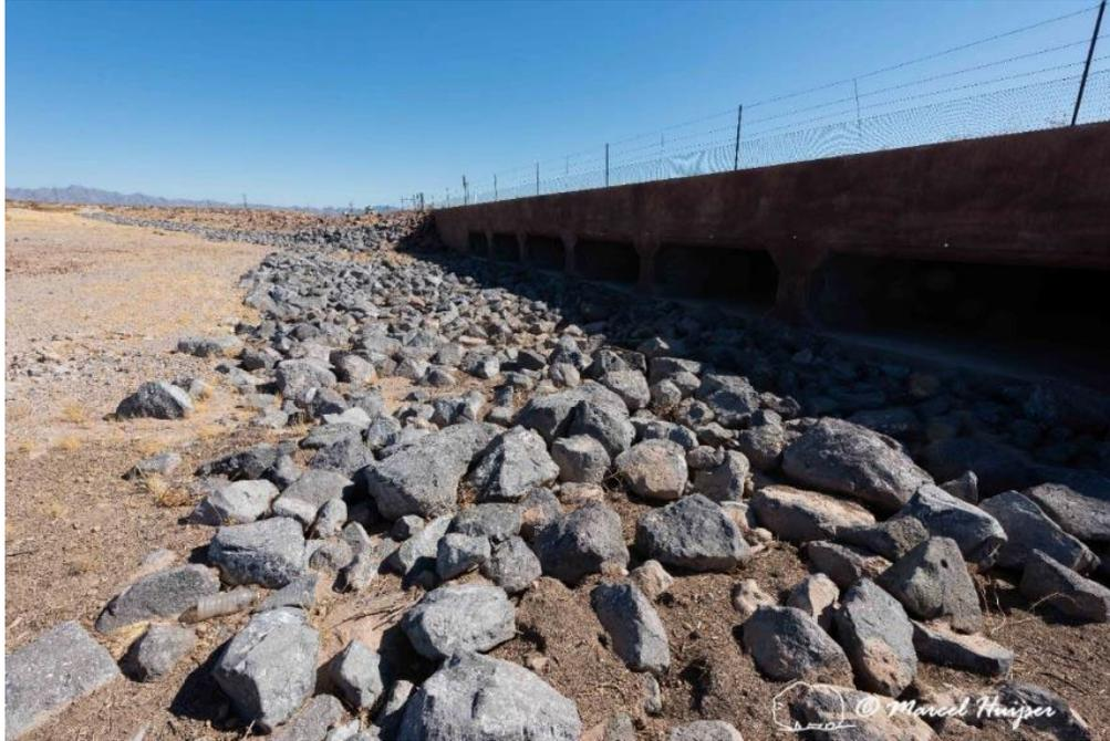
Riprap in front of culverts to reduce erosion, I-11, near Boulder City, Nevada. While beneficial to combatting erosion and sedimentation issues, the size and placement of the riprap most likely results in a substantial barrier to Mojave desert tortoises.
