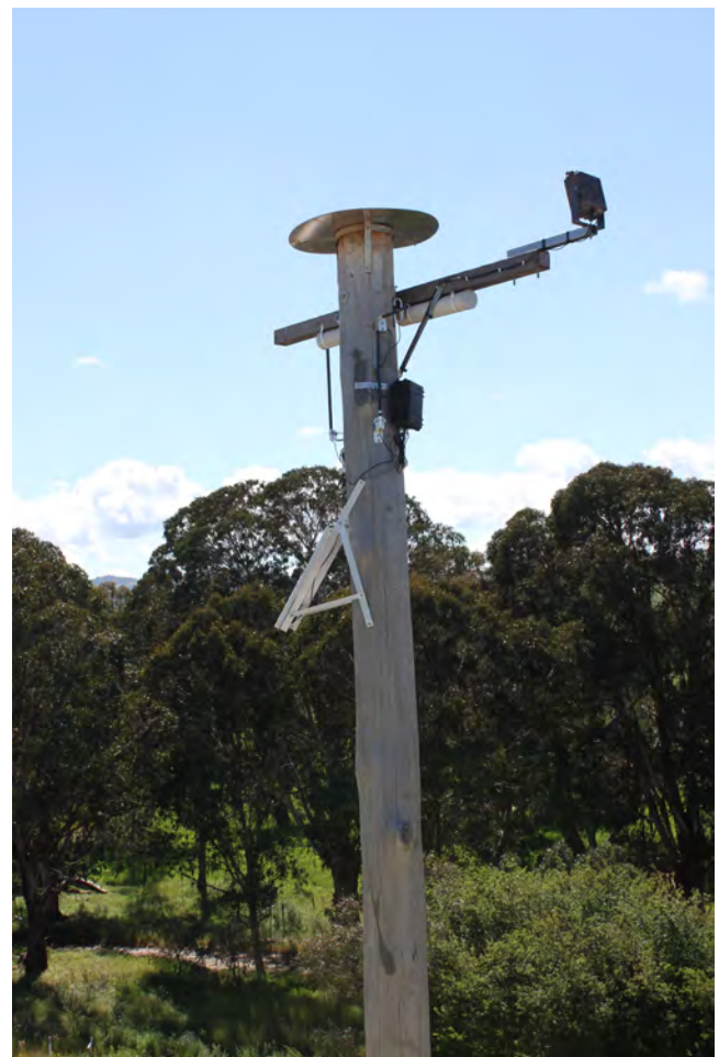
Glider poles are installed on the verges of linear infrastructure or in the centre median at locations where the size of the gap in tree cover exceeds the glide distance of gliding animals. This close-up shows the cross-arm or launch platform at the top of a glider pole, along with cameras and solar panels to evaluate use. The metal shield on top of the pole and the pipe under the cross arm provides shelter from aerial predators. The cross-arm points towards the trees on the opposite side of the infrastructure, thereby decreasing the size of the gap to be crossed. © Rodney van der Ree
