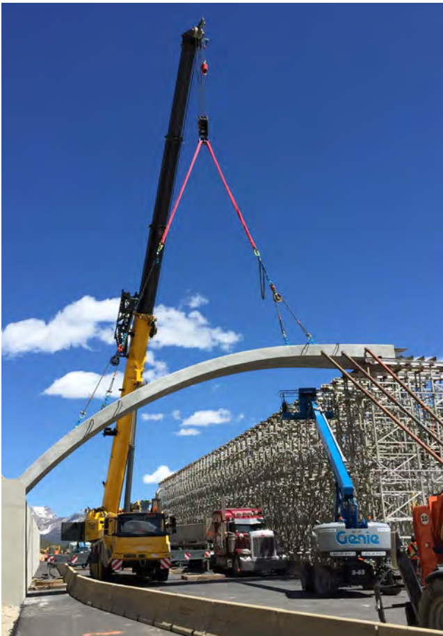
Construction of an overpass over Interstate 90 on Snoqualmie Pass, Washington, USA. Spanning six lanes of traffic, this large overpass is just one piece of a multi-phase, multi-decade effort to restore connectivity in the Cascade Range. Other elements include a 330 m elevated stretch where wetlands and creeks flow beneath the highway, and numerous expanded culverts. Monitoring has documented around 4,000 successful wildlife crossings per year. © Terry McGuire
