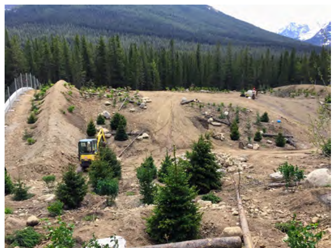
Overpass construction in progress that includes natural surfaces, vegetation variations and design elements to reduce noise and light disturbances to provide favourable conditions for a diversity of species to cross the Trans-Canada Highway, Banff National Park, Alberta, Canada. © Terry McGuire
