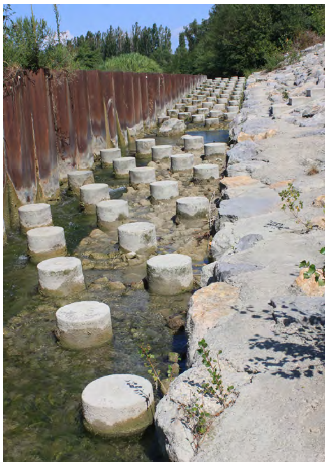
Fish ladder on the Roubion River near Lyon, France. This structure was built in 2011 to provide passage for fish around a weir in place since 1964, originally built to protect downstream infrastructure from flood damage. The ladder and ledges were designed for eels, numerous fish and beaver. © Rodney van der Ree
