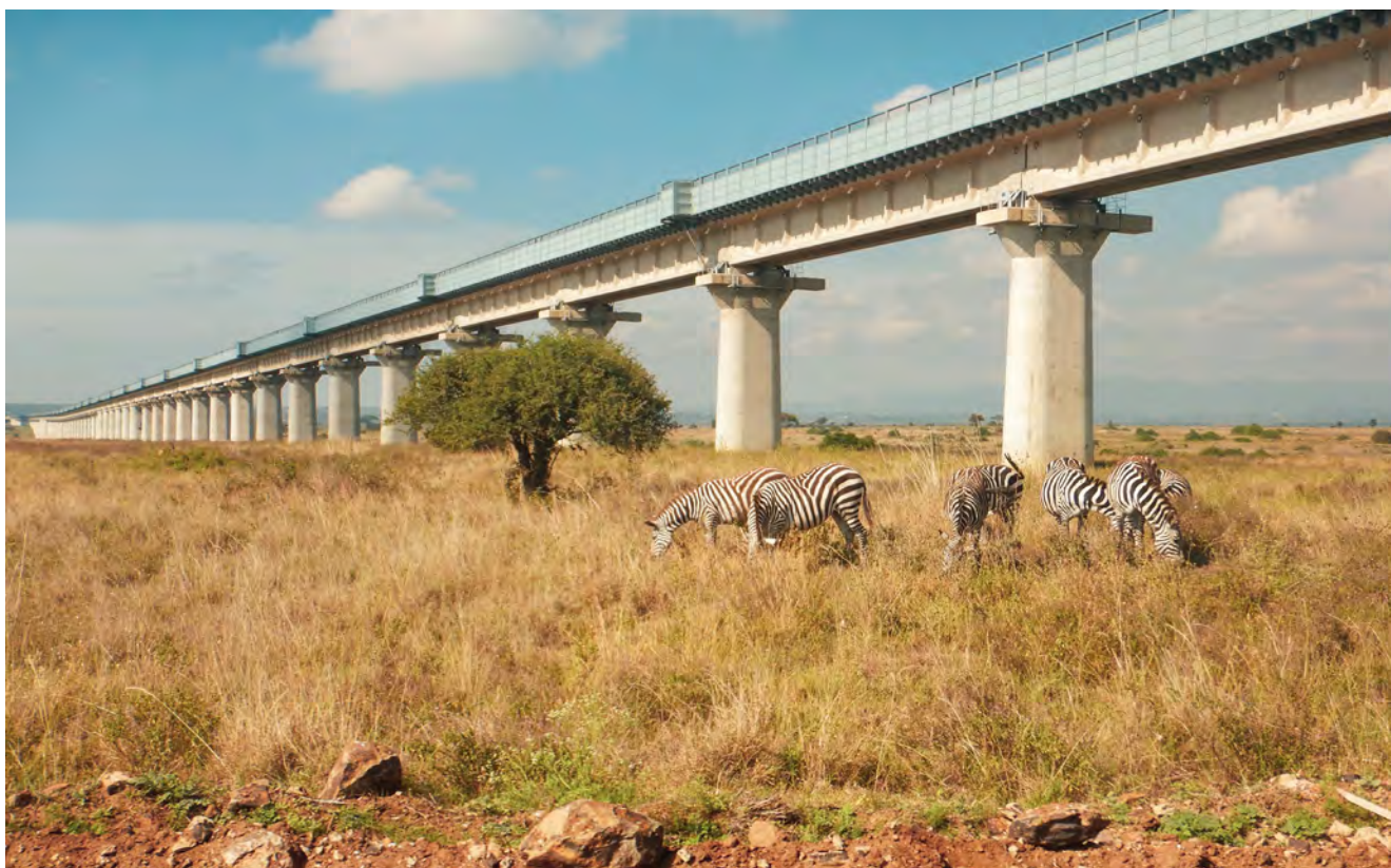
A herd of plains zebra ( Equus quagga ) graze below the Nairobi-Mombasa Railway. Bisecting Nairobi National Park, the rail design allows for wildlife movement under the tracks, but avoidance of the protected area was not taken into consideration. Consequently, the impacts of construction, maintenance and rail effects such as noise, vibrations and movement, are now pervasive. © Martin / Adobe Stock
