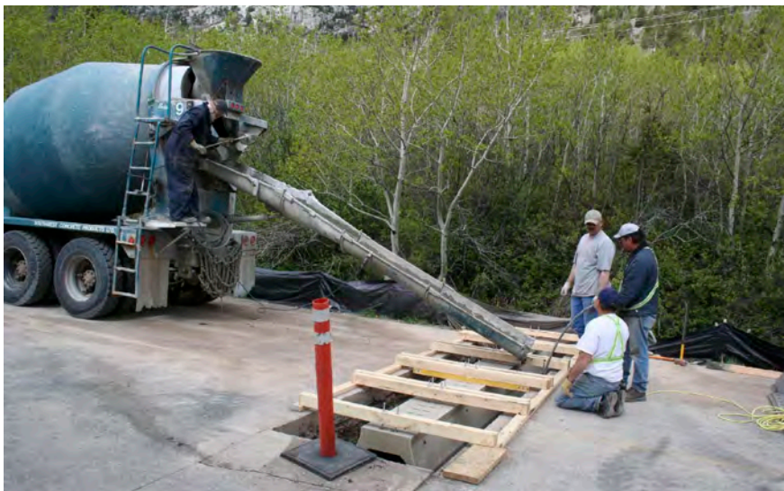
Construction of a salamander-friendly underpass tunnel in Waterton Lakes National Park, Alberta, Canada. © Cyndi Smith, Parks Canada
