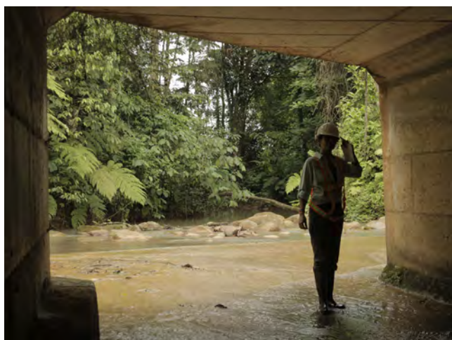
A technician stands in a highway underpass incorporating design for free stream flow and ledges for dry passage by wildlife. © Daniela Araya-Gamboa/ Panthera
