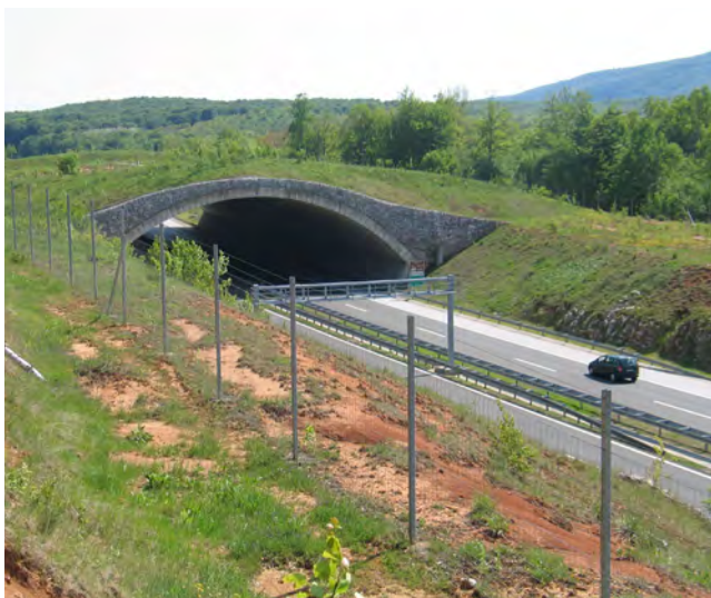
Wildlife crossing structures can be even more effective when integrating directional fencing to funnel animals to the safest passage and reduce rates of collisions with vehicles. Left: The 100 m wide Dedin green bridge' with directional fencing in the foreground was constructed along with 43 viaducts and tunnels on the highway stretching 68.5 km from Zagreb to Rijeka in Gorski kotar (Croatia). © Djuro Huber; Right: Underpass on US Highway 93 with directional fencing on the lands of the Confederated Salish and Kootenai Tribes (CSKT) of the Flathead Reservation in Montana, USA © Luca Guadagno
