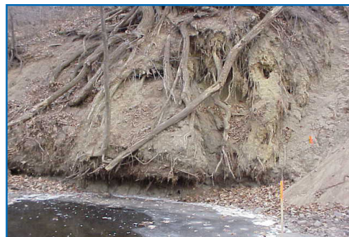
Example of soil erosion along a creek.
