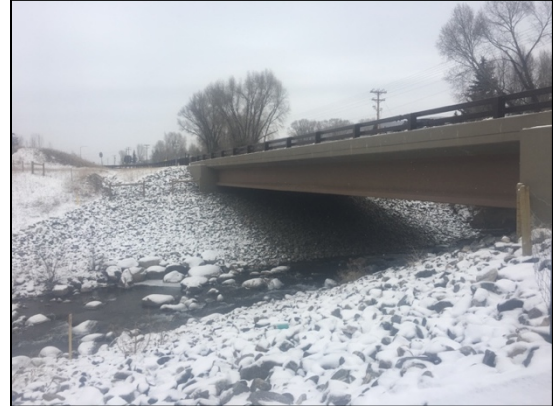
Riprap slopes under Lake Creek
