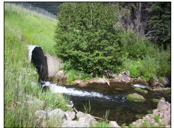
Existing pipe culvert (outlet) at Red Sandstone Creek
