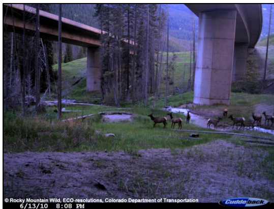
Elk under divided span bridge at MP 185.5
