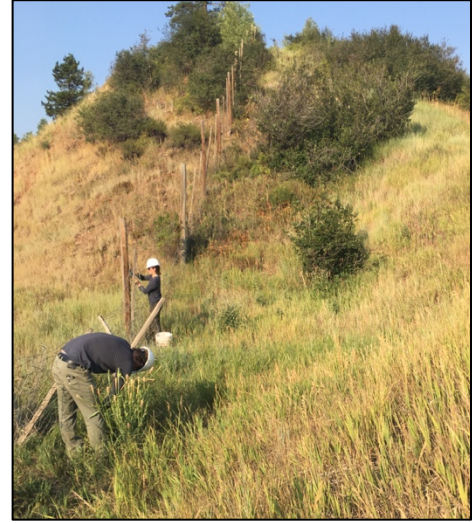
USFS removal of a section of redundant wildlife exclusion fence.
