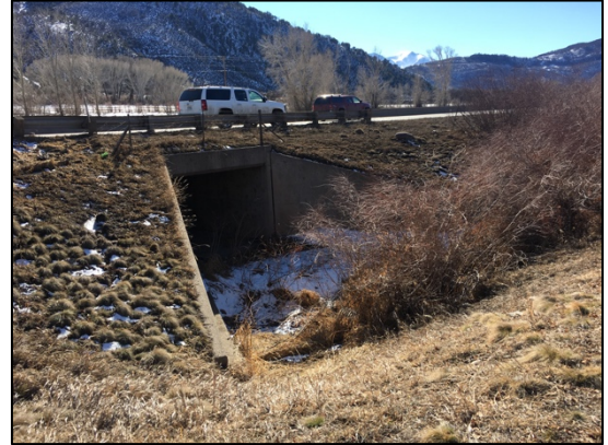
Box culvert at MP 22.1
