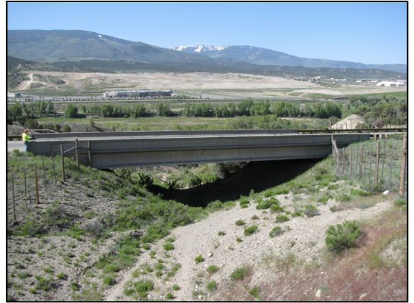
Double span bridge at MP 143.1
