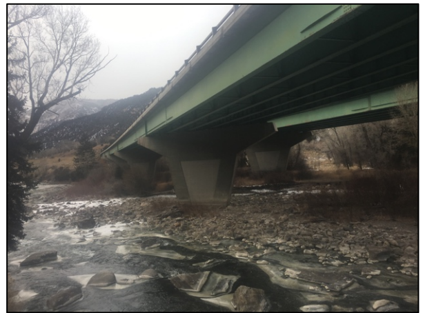
Multi-span bridge over the Eagle River at MP 154.0
