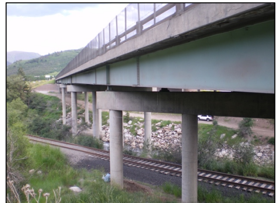
I-70 bridge over US 6, railroad and the Eagle River at MP 168.9
