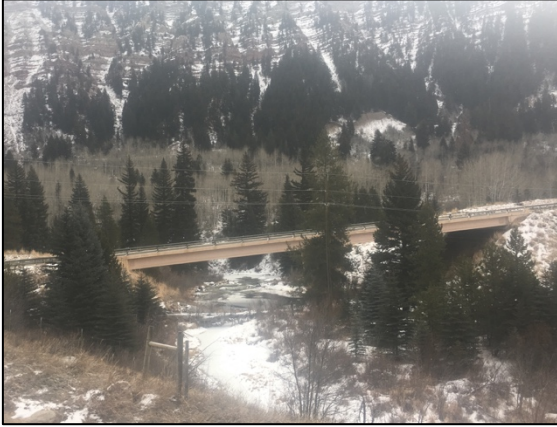
Eagle River bridge (MP 148.3)
