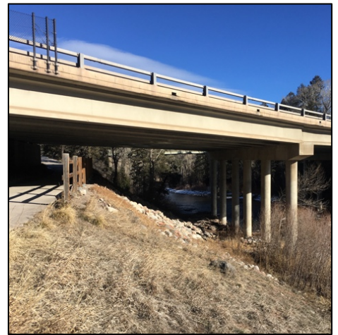
Riprap bank under bridge at MP 21.1
