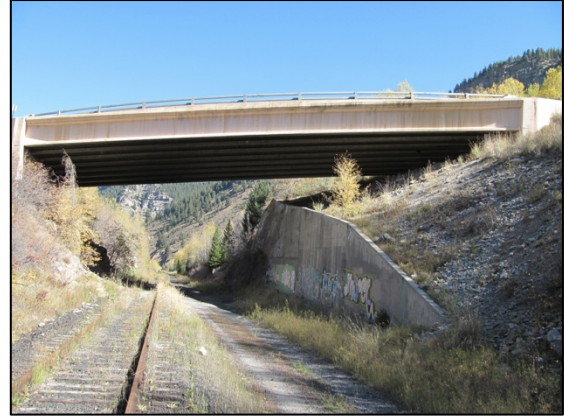
Railroad bridge (MP 148.4)
