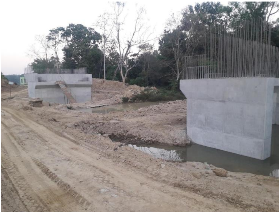
Figure 4: Wildlife underpass abutments awaiting girders and then excavation on Chittagong – Cox’s Bazar railway project. Final dimensions: 4.5-m height, 30-m length. Credit: Asif Imran.
