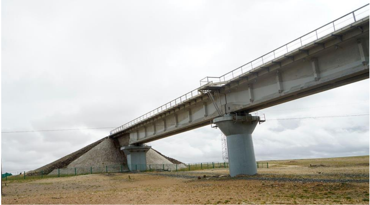
Figure 14: The Wubei Underpass allows for Tibetan antelope to pass underneath the railway. The four underpasses are the only means for Tibetan antelope to cross the railway, as the entire railway is fenced. Of the four underpasses, the Wubei underpass is used the most by Tibetan antelope. Credit: Wenjing Xu.
