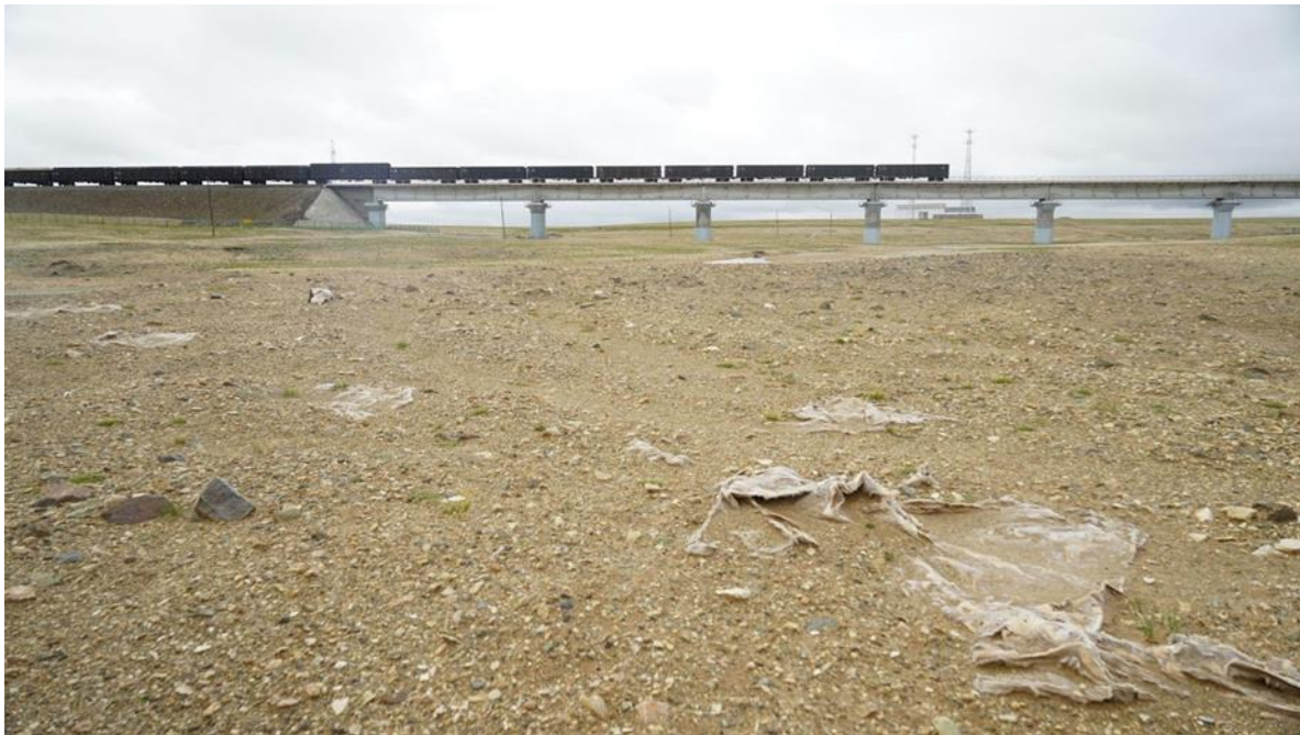
Figure 13: The Qinghai-Tibet Railway in Central China. The long-distance migration of Tibetan antelope is directly affected by the Qinghai-Tibet Railway. Four major crossing structures were constructed for the Hoh-Xil area, including the Wubei underpass. Credit: Wenjing Xu.
