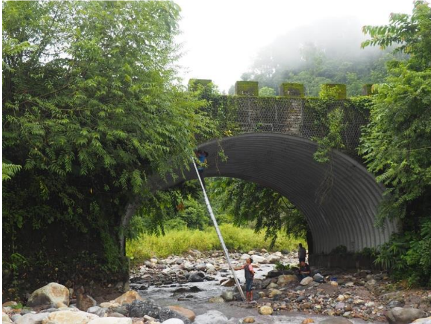
Figure 7: Wildlife underpass designed primarily for elephant passage on the NH2 road (Raidak-Lhamoizingkha). Credit: Karma Chogyel.
