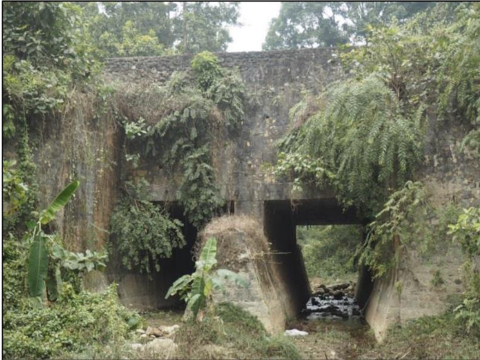
Figure 19: An existing twin-cell minor bridge currently exhibiting limited wildlife passage potential. This structure is planned for replacement with a 6-m high and 16-m wide single span minor bridge. Credit: Anthony P Clevenger.
