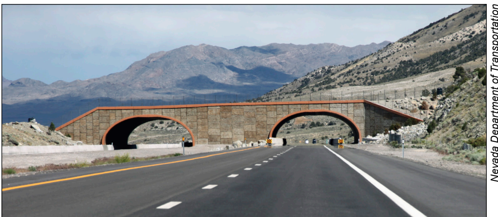
Figure 10—Mechanically stabilized earth end treatment used on wildlife overpasses across I-80, near Wendover, Nevada.
