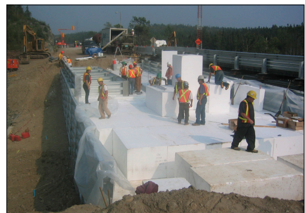
Figure 13—Expanded poly-styrene geofoam used in construction.
