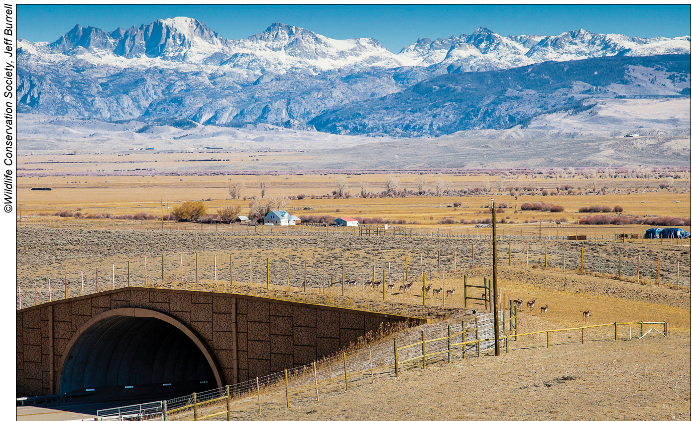
Figure 3—Pronghorn antelope using Trapper's Point wildlife overpass across U.S. Hwy 191, near Pinedale, Wyoming. This overpass was placed at a migration route for pronghorn, enabling it to be used by migrating pronghorn within days of its completion.
