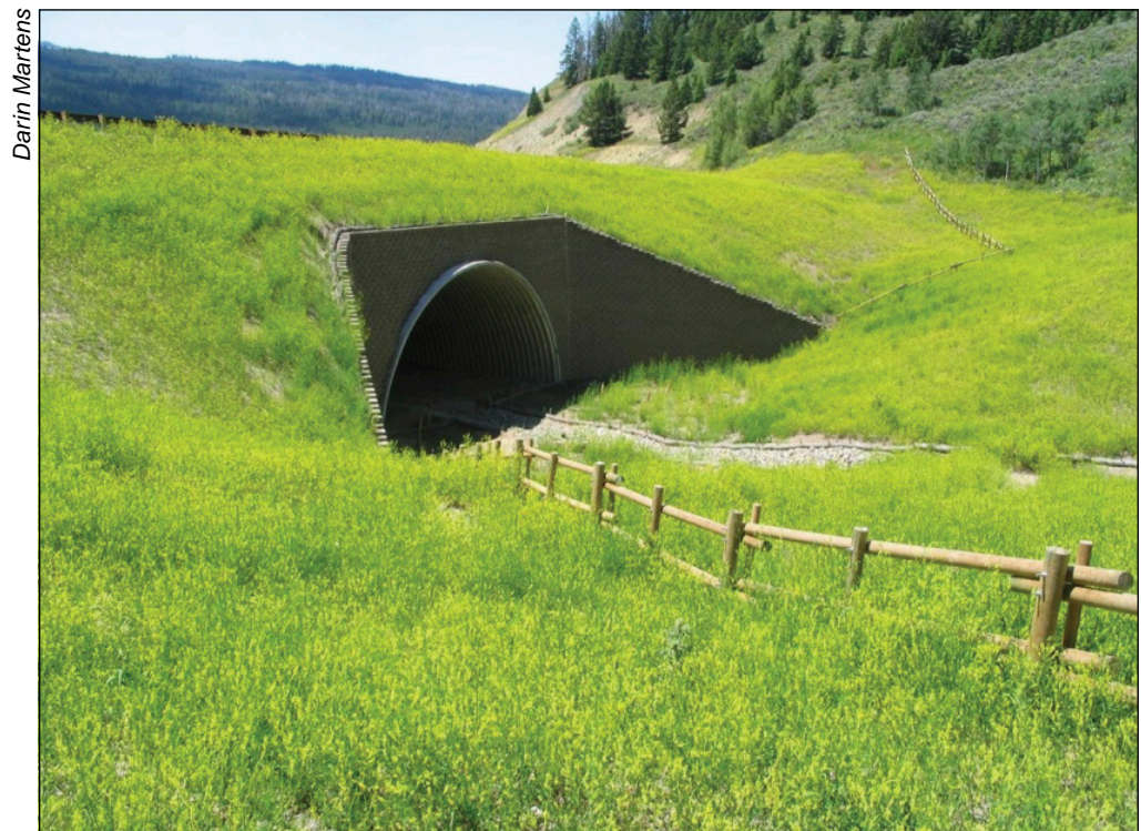
Figure 9—Togwotee Corridor reconstruction, 50' diameter arch wildlife crossing structure during the flowering of yellow sweet clover ( Melilotus officinalis ).
