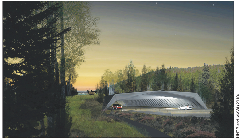
Figure 3. Stacking two worlds: a pillar-free and modular integrated wildlife overpass design constructed using precast concrete.
