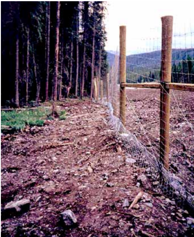
Figure A1: A 10.2 cm (4 inch) square mesh, metal woven fence that is 2.4m high (~8 feet) with buried apron along the Trans-Canada Highway in Banff National Park (Phase 3-A) (© Tony Clevenger).
