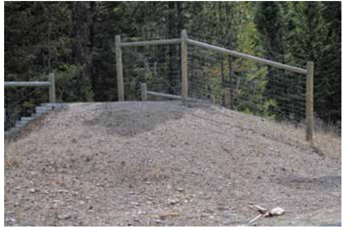
Figure A2: This jump out or wildlife escape ramp was constructed on U.S. Highway 93 in western Montana as an opening created in the highway fencing to allow wildlife caught on the highway side of the fence to jump out to safety (© Rob Ament/WTI).
