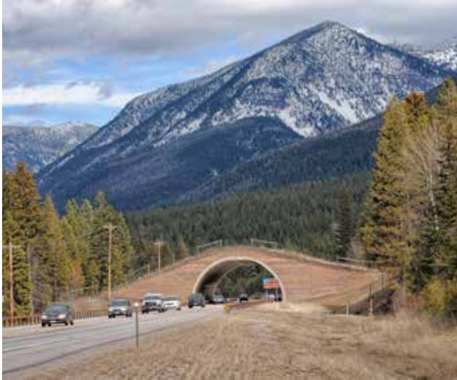
Figure A3: Wildlife overpass on U.S. Highway 93 on the Flathead Reservation in western Montana (© Rob Ament/WTI).
